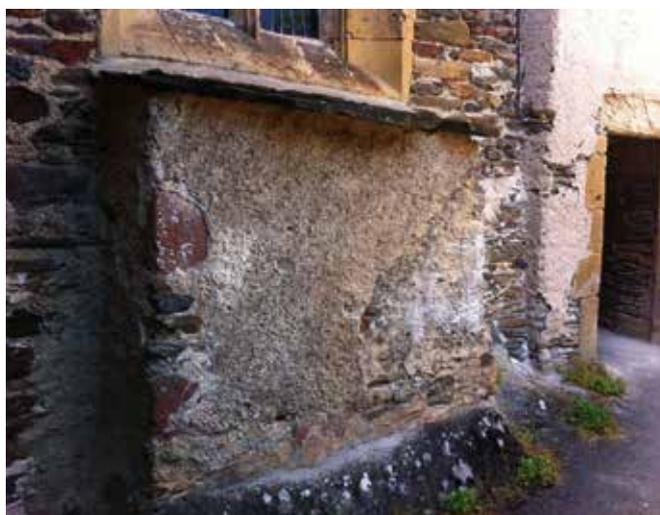
FIG. 24C. VUE DE LA MAÇONNERIE DE PROTECTION CONSTRUITE APRÈS LE PERCEMENT
