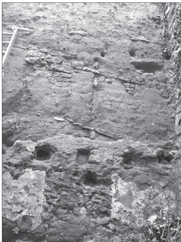
FIG. 10. DANS LA PARTIE INFÉRIEURE DU MUR EN BAUGE, MOTTES FAÇONNÉES MANUELLEMENT. MONTAGNAC (Hérault). Cliché C.-A. de Chazelles.
