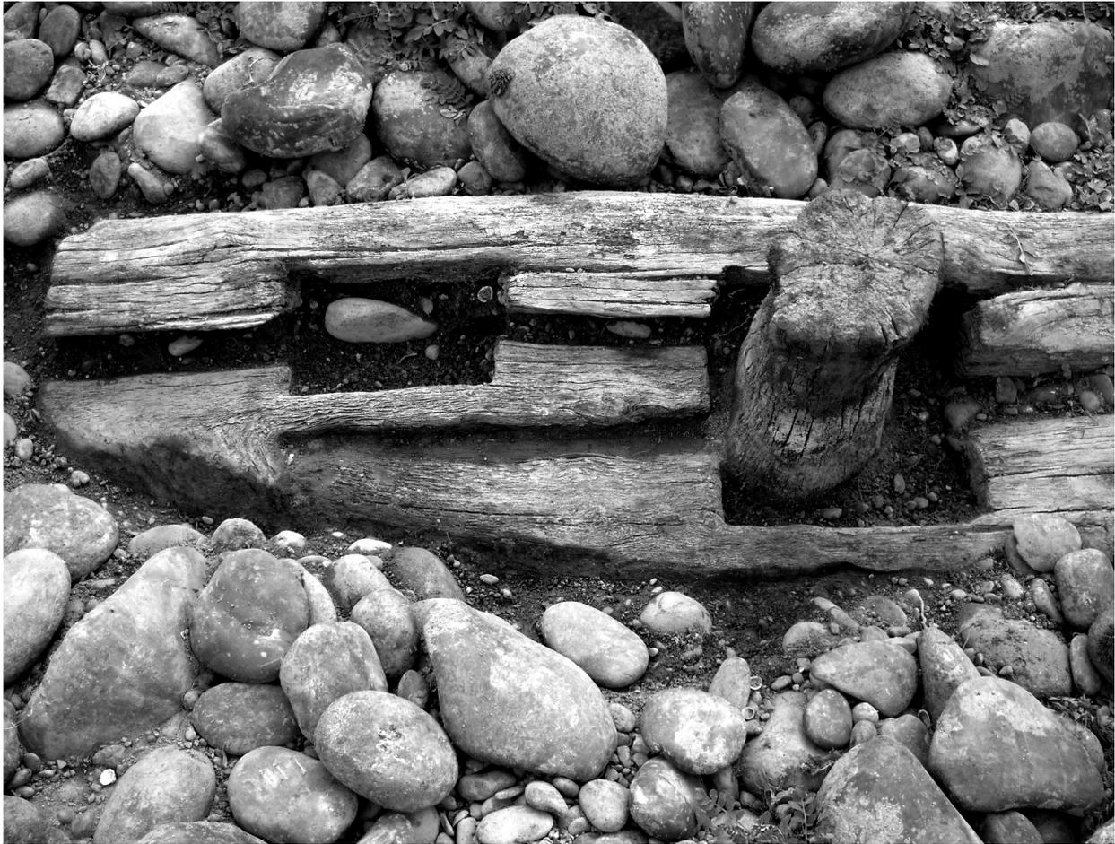
FIG. 12. MARQUEFAVE. DIGUE-BARRAGE DU MOULIN DE SAINT-HYPPOLITE. Mortaises et pieu P 128. *Cliché M.-T. Tinet-Lassure.*
