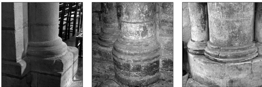
FIG. 2. PROFILS DE BASES À SCOTIE APLATIE.
